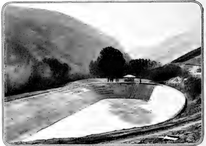
By lining a useless old pond with concrete five million gallons were added to the city's storage water supply
